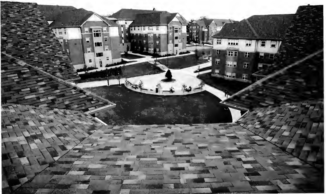
Foreground: Roof of Suite 316 on Maple West; background: Putt Hall, left, and Delaney Hall The view is from the northwest corner of Maple and Eleventh streets, looking northeast
